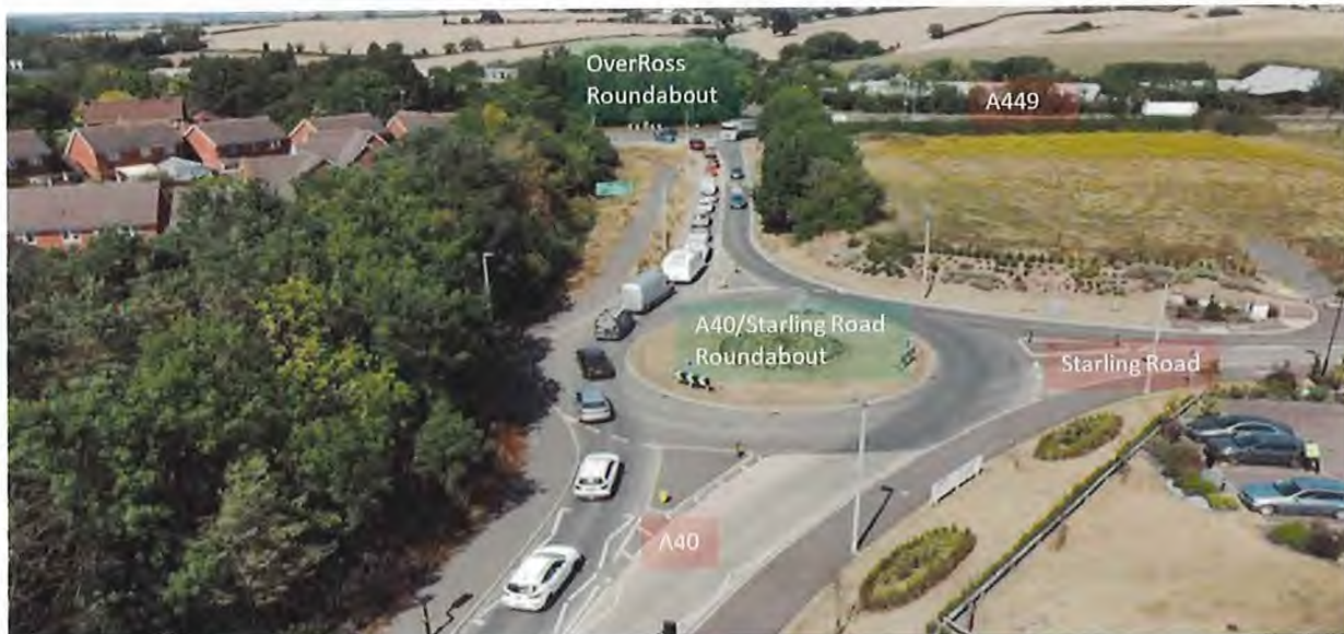
Picture 1 – A40/Starling Road and OverRoss roundabouts
